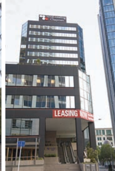
4 The Shortland Centre WHK Gosling Chapman Tower, 51-53 Shortland Street Ji Ah Lee
